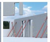
At least two mounting anchors are required for each wall element when installing the concrete wall elements.
