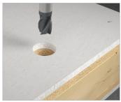
Machine creation of the precise installation opening of Ø 38 mm.
