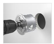
Create installation opening Ø 68 mm with KAISER cutter (e.g. EXPERT, Art.-No. 1082-30).
