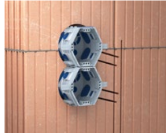
Insert the UP 1 one-gang or one-gang junction box with ribs.
