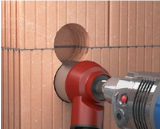
Make the installation opening Ø 82 mm with the diamond grinding crown (Art. No. 1088-02).
