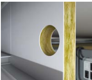
Create an installation opening of 50 mm in diameter.
