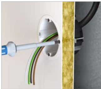
The box is inserted into the component opening and fastened with the screws.
