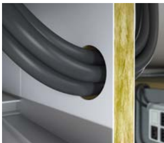
Feed the cables through the opening in the component.
