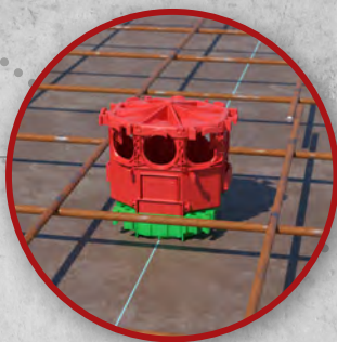
Simply insert the conduits into the prepared openings
