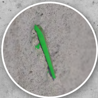
Signal bristles for easy location of the boxes after removing the formwork
